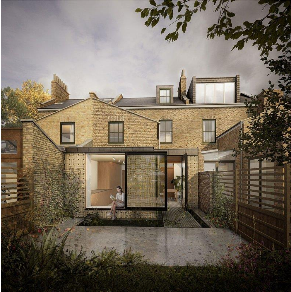
The basket weave pattern was conceived to break down the massing of the rear elevation.
